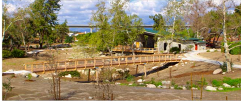
Walnut Creek Nature Park Improvements
