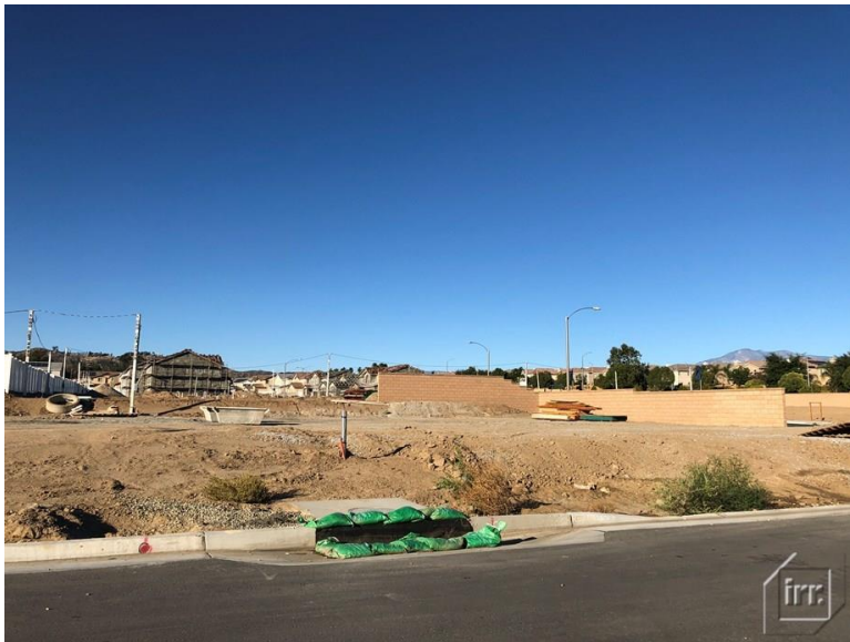
Community Facilities District No. 2015-3 (Athens) N/O Eucalyptus Ave., W/O Nason St. Moreno Valley, California
