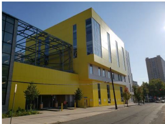
External View of Project Facilities
